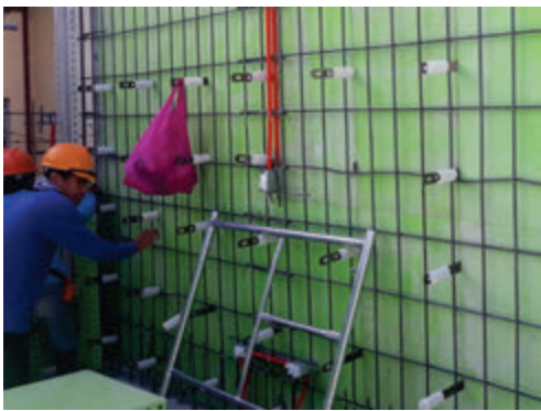
MEPFS are Installed. Foam is wrapped around the flat ties for easy pull out & reuse
