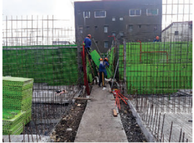
Erection of wall on ground slab
