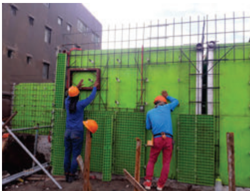
Blockouts for openings
