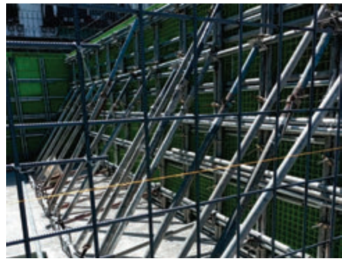
Two-sided wall fully installed and aligned
