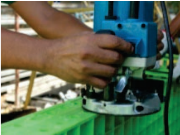
Use rotor for notching of Plasmform
