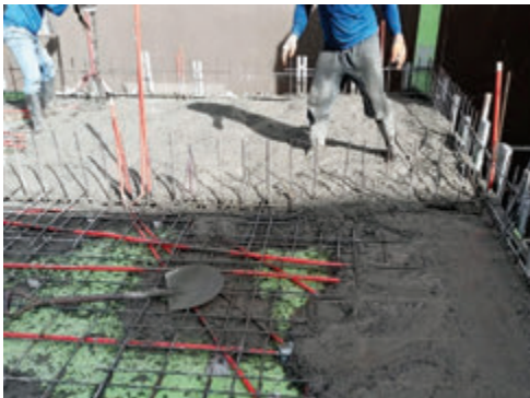
Monolithic concrete pouring of wall and slab
