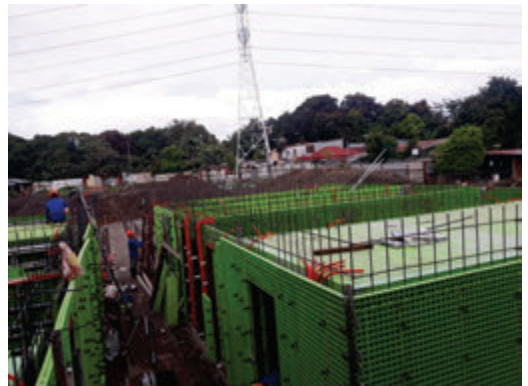
Wall and slab formworks with MEPFS
