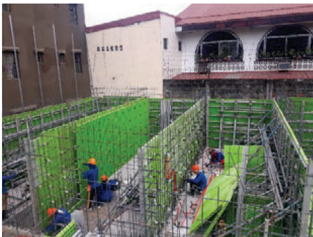
Installation of flat ties to hold the forms on both sides
