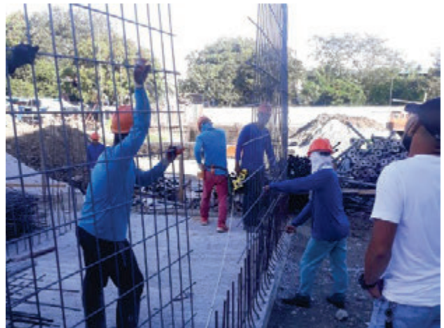
Continuation of installation of steel mat for Wall
