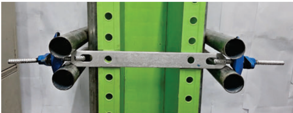
Full Assembly of manual handling wall form using flat tie
