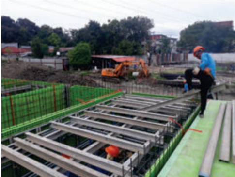
122 Aluminum Beam used for joist for Slab Forms installation
