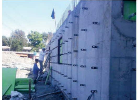
Smooth concrete finish is achieved and can be finished with skim coating.
