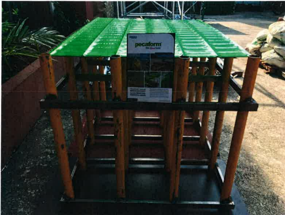
Pecaform Load Test Set-Up
