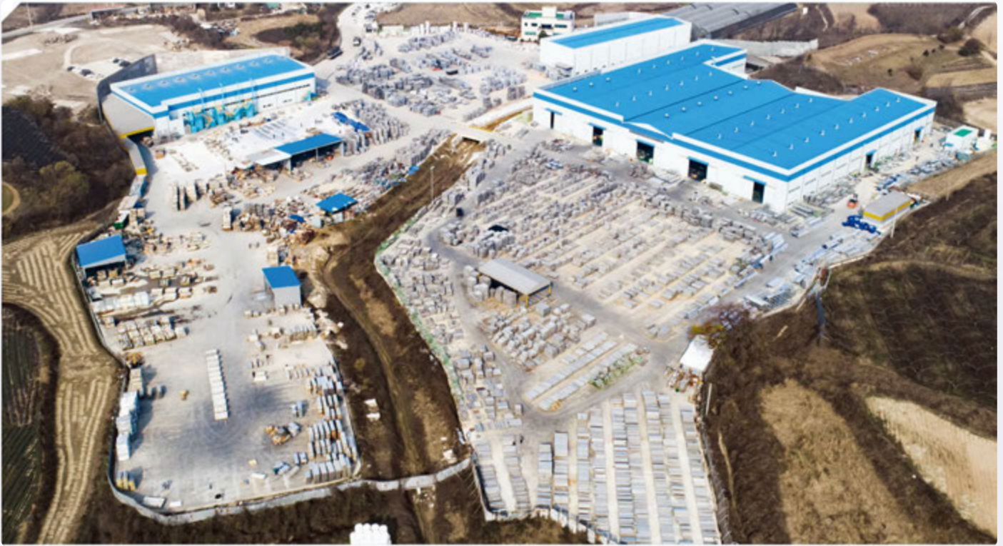
View of the formwork factory
